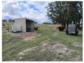
Thanks again to Kelvin, Geoff & Tony who have installed a 1000L IBC next to the shed and plumbed it up to catch water from the shed roof and fitted a discharge to the IBC to match up with our pump. So we now have the option to run the pump from the IBC whenever there is enough water in it. It is already half full. A side effect of the new shelter is that the site is also now much better organised and better looking.
